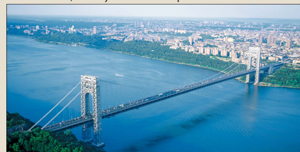
THE GEORGE Washington Bridge is a double-decked suspension bridge spanning the Hudson River, that connects the Washington Heights neighborhood of Manhattan in New York City with the borough of Fort Lee in New Jersey. The bridge is named after George Washington, the first president of the U.S..
